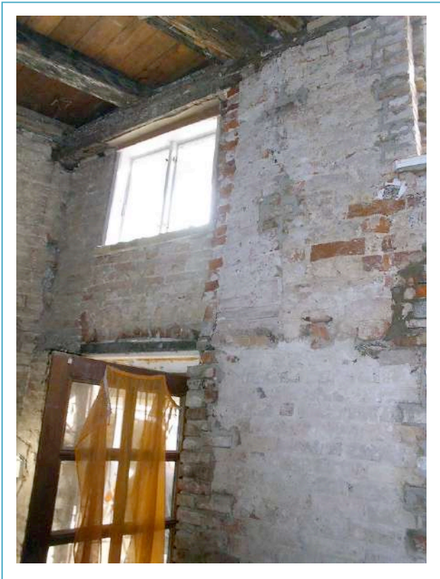
Image No. 15, street facade with head rail of the former timber frame construction, © LAKD M-V, LD, Jan Schirmer
