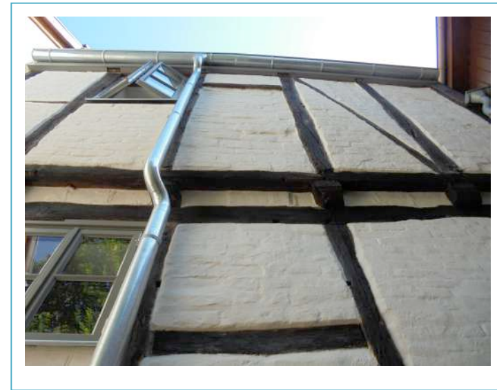
Image No. 18, courtyard facade after sanitation, 2016 © LAKD M-V, LD, Jan Schirmer
