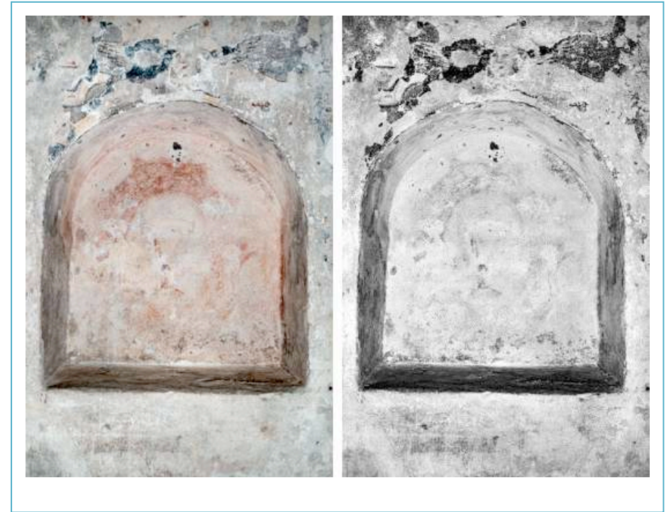
Image No. 10, Detail of the west wall during its conservation. Scattered photograph and IR photograph (~ 900nm). Photograph: Rapolas Vedrickas, 2019.
