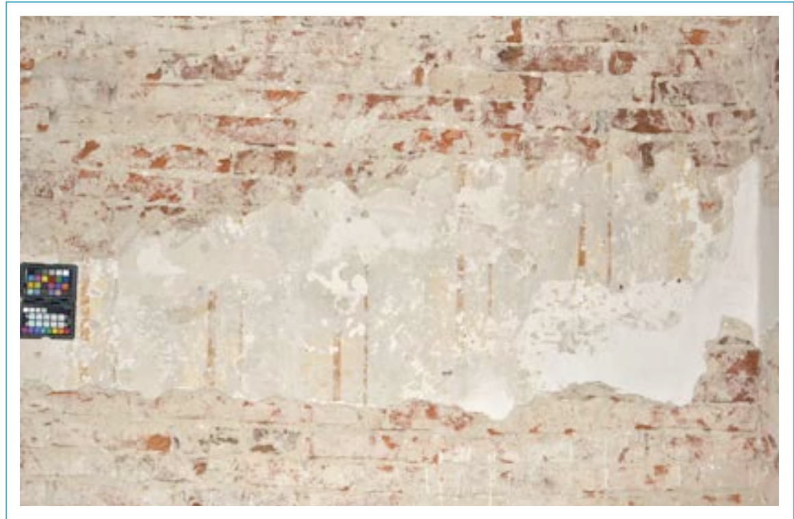
Image No. 11, Ground floor – wall polychromes, photo by Marta Boguta
