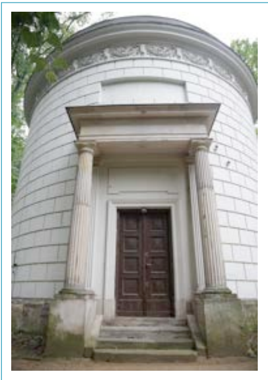
Image No. 2, Elevation before the conservation, photo by Marta Boguta
