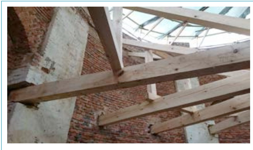
Image No. 8, Roof truss during the conservation, photo by Maciej Czyski
