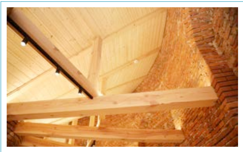
Image No. 26, Roof truss after the conservation, photo by Paweł Czarnecki
