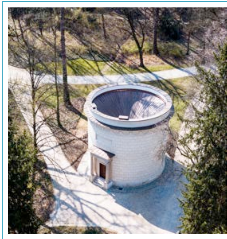
Image No. 17, Aerial photo of the building, photo by Volatus Media
