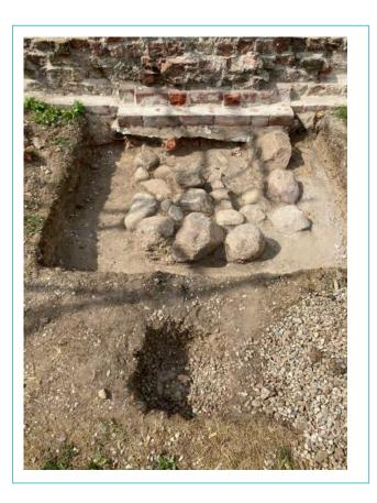
Image No. 12, Field stone foundation of Valdemar's Wall and position of the drainage in front of the wall, August 2020. © ALSH
